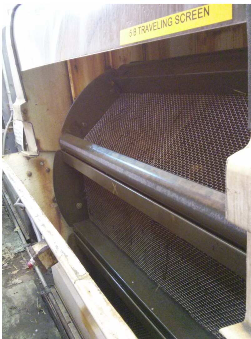
Figure 9-1: Schiller Station's Unit 5 Intake Screen
