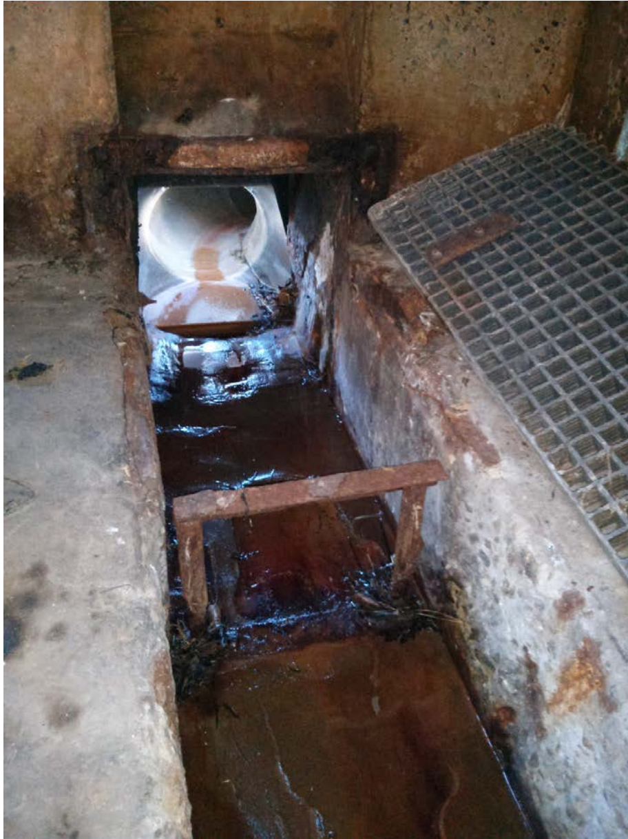
Figure 9-3: Unit 4 Fish Return Trough
